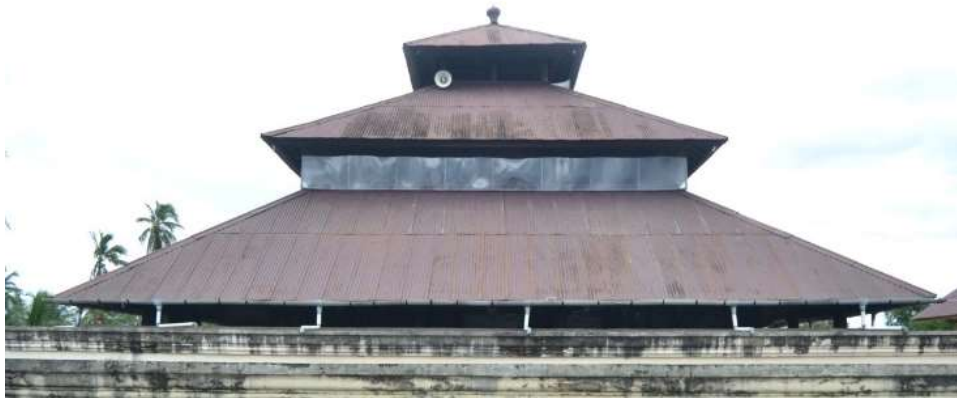
Figure 2. The Roof Condition of The Mosque (source: Putra, 2018)
